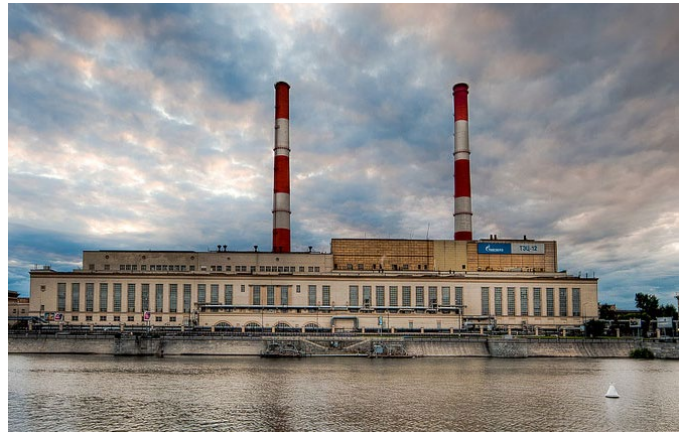
Gazprom facility on the Moscow River.
